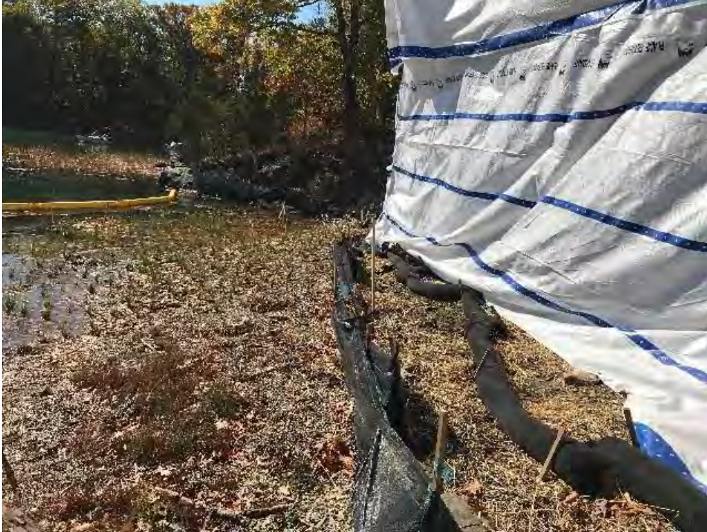
Fig 11: Toe of the slope below the cable house at Eversource property/west side of the bay. Viewing south. (10-14-20)
