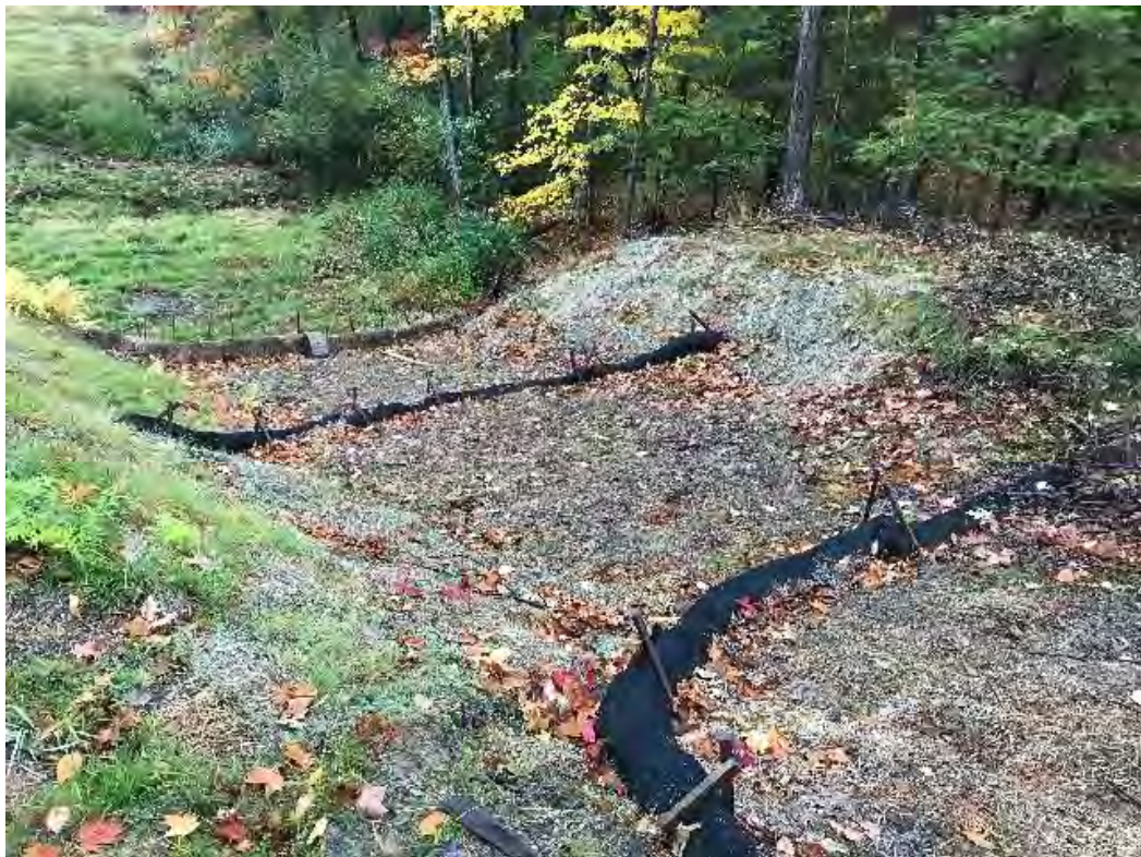
Fig 14: Slope between Strs. 28 and 29. Viewing northeast. (10-14-20)
